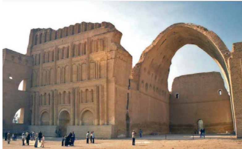
1. Ctesiphon. Raw bricks arch (40 meters high). 4th century BCE (Baghdad, Iran).
